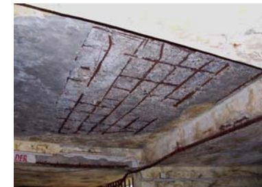
Roof of classroom at ITI Ankleshwar
