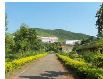
Status of campus maintenance at ITI Vishakhapattanam
